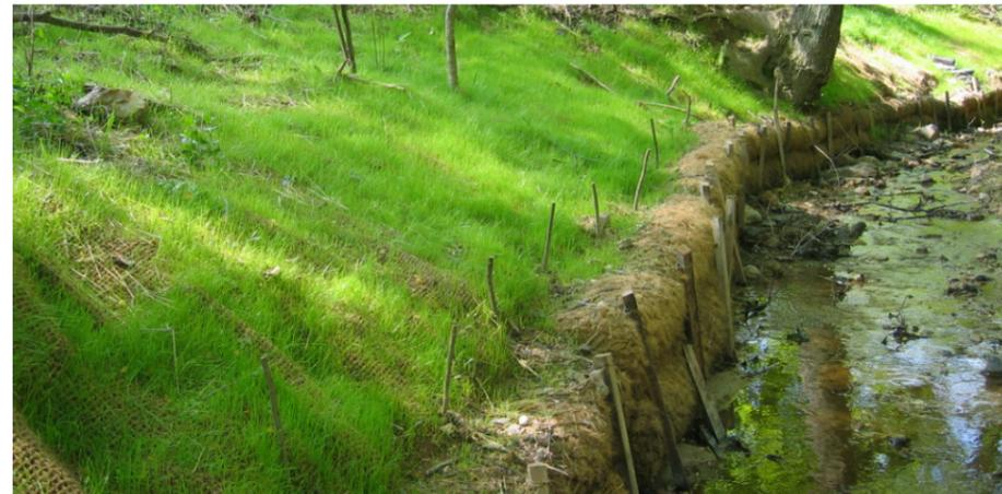
Coir logs installed at the toe of the stream bank. Image courtesy of Department of Environmental Protection Montgomery County, MD.
