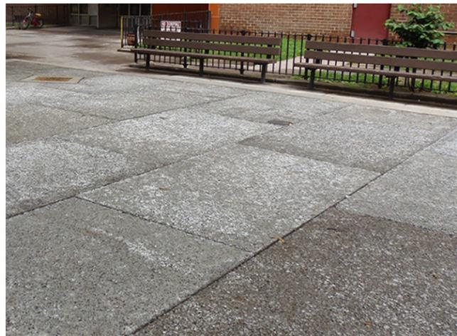
Images of a pervious concrete sidewalk. Courtesy of NYC Department of Transportation.
